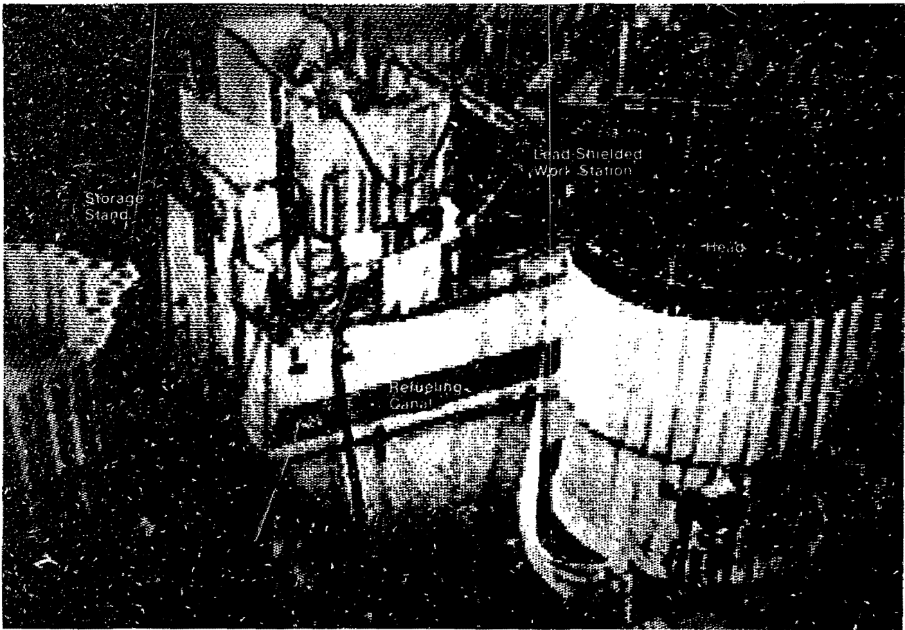
Figure 2. Photo taken from television monitor of the head traveling toward the head storage stand.
